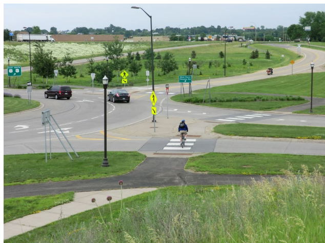
Example of a multi-lane roundabout.
