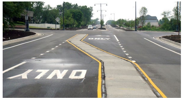
Example of left-turn lanes.
