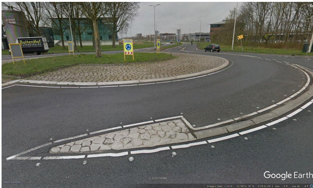
Figure 14. Photograph. Example introduction of the raised lane divider. (30)
