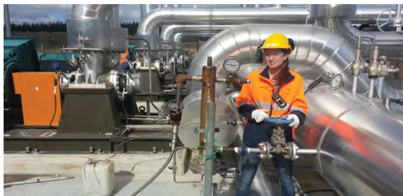
A plant chemist samples silica concentrations from a geothermal injection brine line. Photo credit: Jeff Winick/Allegheny Science and Technology
