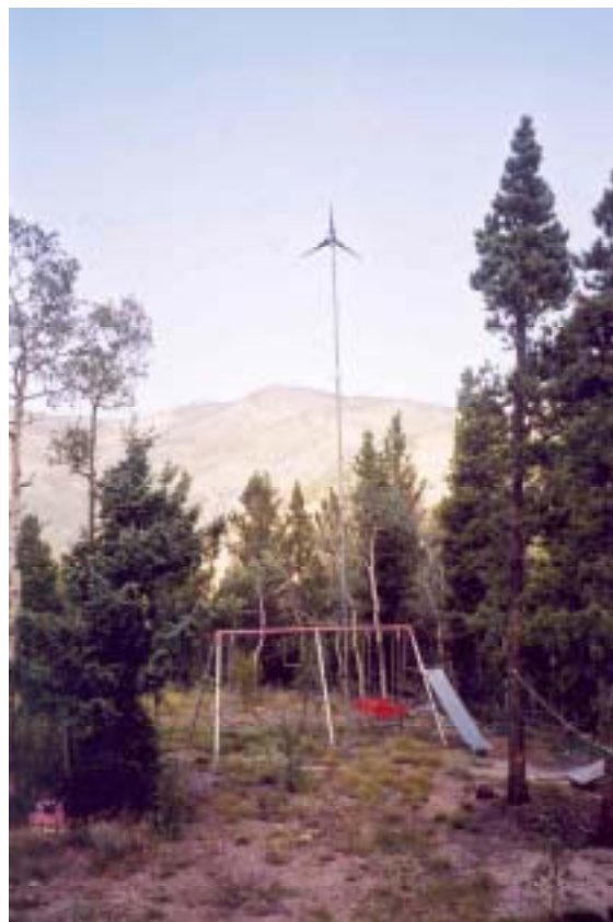
Figure 6.6. WTG on 27-foot tower
