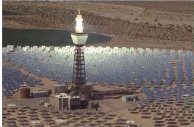
Figure 1: Above, power tower pilot project, pioneered in the U.S. (Barstow, CA) and (left) commercial unit under development by Abengoa called PS10, an 11 MW plant in Sevilla Spain (photo credit: Abengoa Solar). Bottom left, Stirling Dish/Engine, Center SEGS trough plants, Right, Compact Linear Fresnel Reflector.
