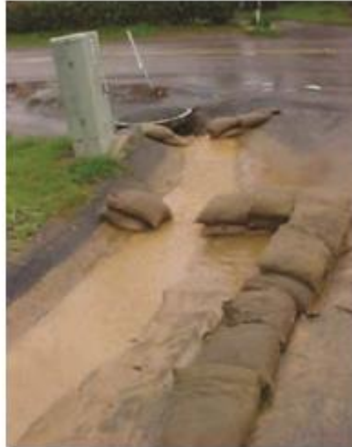
Figure 5. Make sure storm drain inlets are protected
