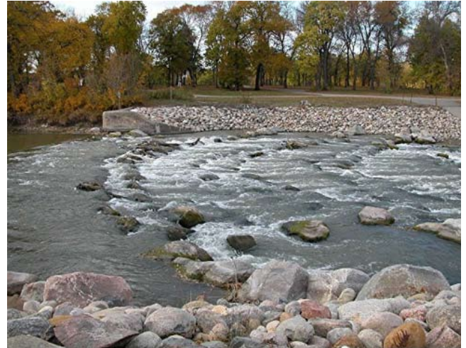
Figure TS14N-15 (a) North Dam on the Red River of the North (ND) before construction; (b) after construction of an engineered channel fishway
