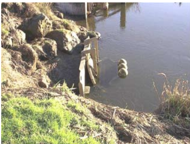
Figure TS14N-28 Self-regulating tide gate
