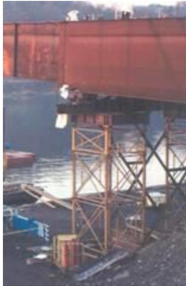
**Figure 7 Photograph of a temporary bent**
