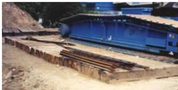
**Figure 6 Photograph of a timber crane mat**
