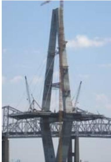
**Figure 17 Photograph showing cantilever cable stayed bridge erection using deck mounted derricks**
