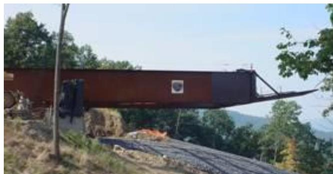
**Figure 11 Photograph showing an I-girder bridge launching**
