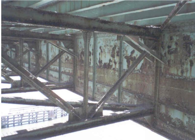
Figure 20. Photo. The area under an open grid deck acting as one large leaking joint.
