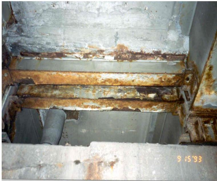
Figure 16. Photo. Steel directly beneath transverse expansion joints that have leaked corrosive runoff from the deck.
