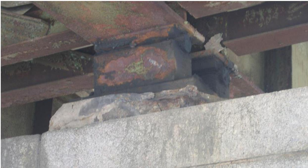
Figure 30. Photo. Corroded bearing.
