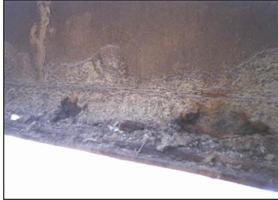
Figure 28. Photo. Heavy corrosion of bottom flange and web due to collection of poulitice.
