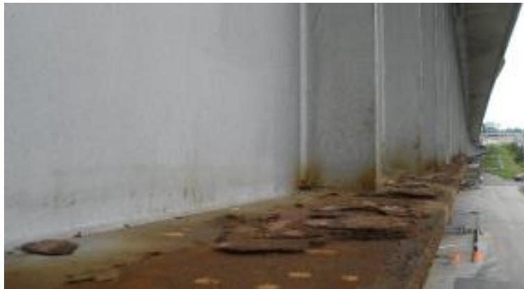
Figure 27. Photo. Corrosion localized to upper surface of lower flange, the rest of the bridge is fine.
