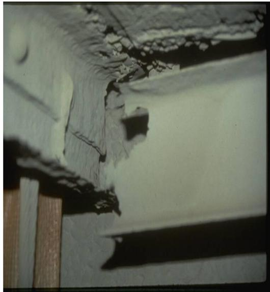
Figure 1. Photo. Photograph of a severed connection due to corrosion.
