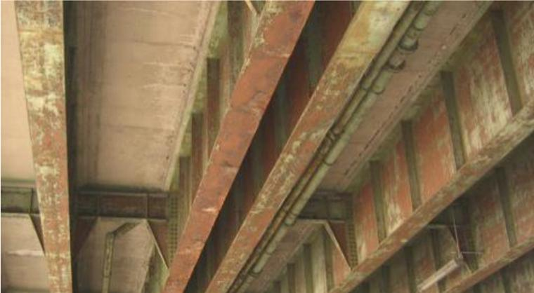
Figure 19. Photo. Closely spaced girders lead to difficult access for maintenance activities.
