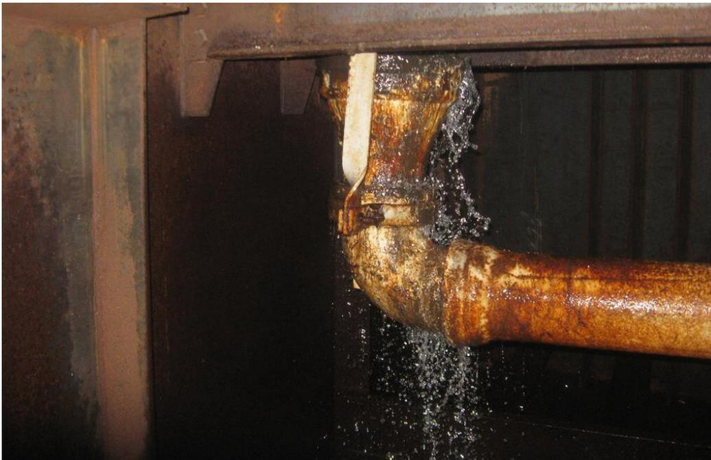
Figure 22. Photo. Clogged drain leaking water onto superstructure.
