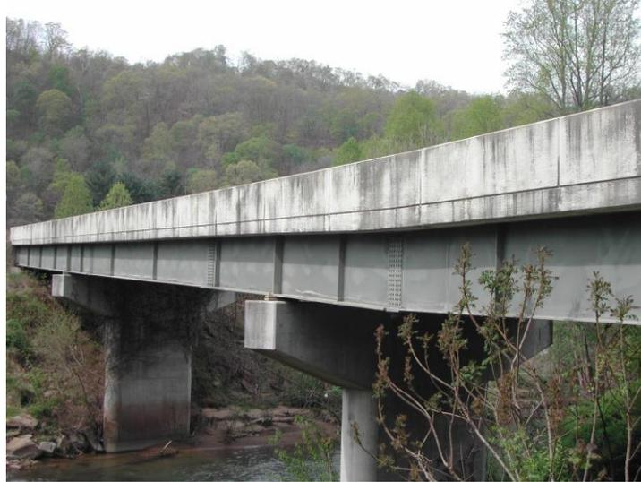
Figure 14. Photo. Bridge in West Virginia with a single-coat inorganic zinc-rich paint system after 25 years.
