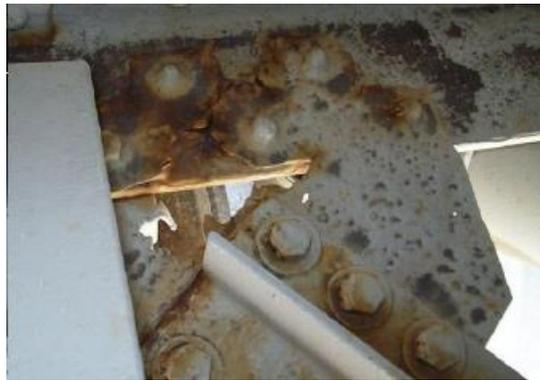
Figure 38. Photo. Corroded lateral gusset plate detail.
