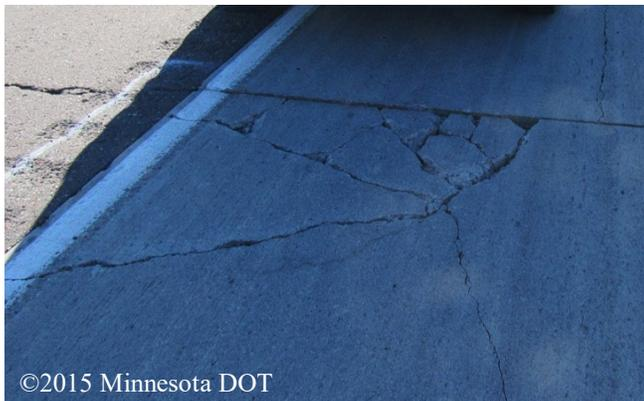
Figure 3. Corner-cracked panel adjoining thermally cracked asphalt shoulder in 5-inch (125 mm) unbonded overlay along TH-53 in Minnesota.
