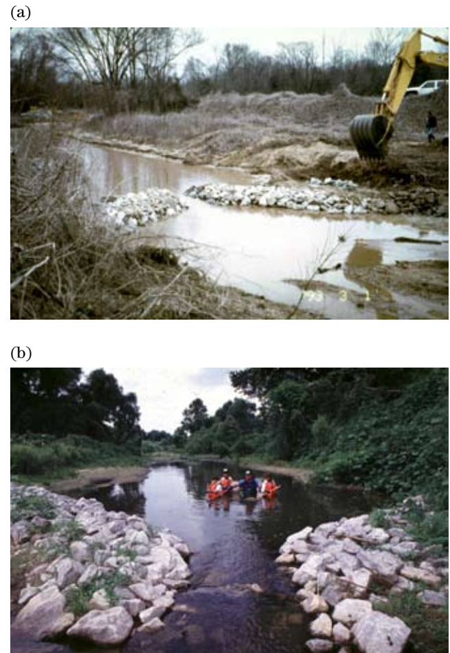
Figure TS14B-15 Scour associated with low stone weir
