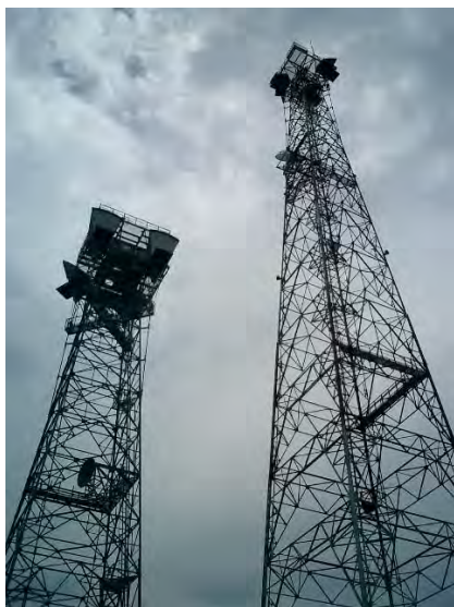
Figure 7-7. Steel tower structures requiring line-line intersections to compute center coordinates based on coordinates observed on each tower leg
