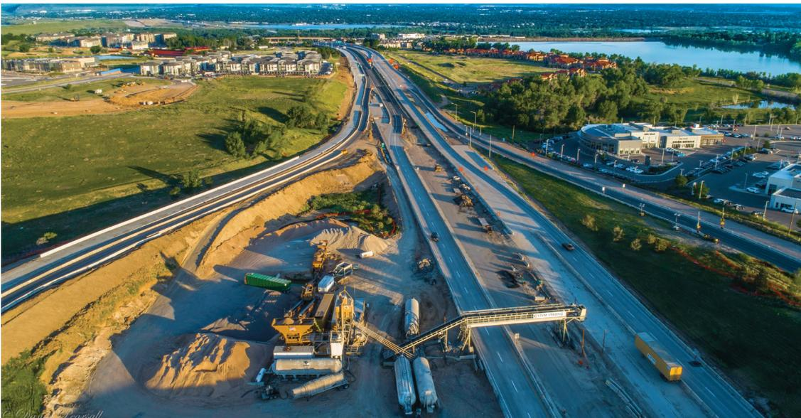
*Figure 2. Crushing plant used to produce RCA for use in new RCA concrete pavement on C-470 in Colorado*
