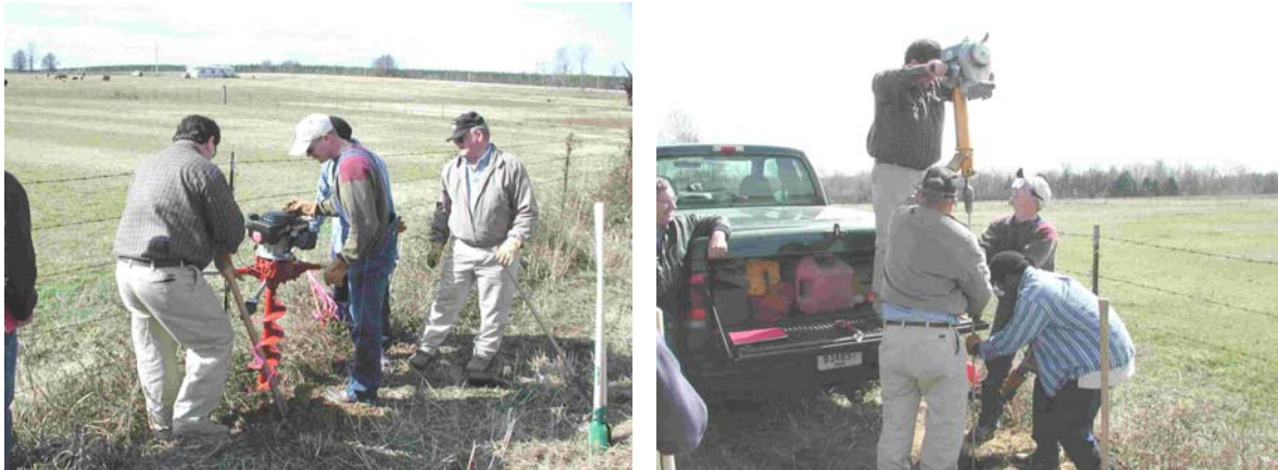
Figure 8-11. Setting deep-driven bench marks (Memphis District & 3001, Inc.)
