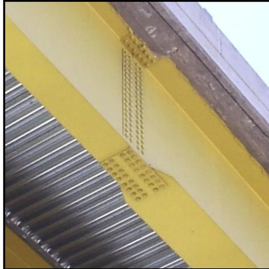
**Figure 2 Photograph of a Steel Plate I-Girder Field Splice at a Flange Width Transition**
