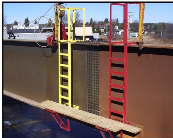
**Figure 10 Photograph of a Girder Web Splice**
