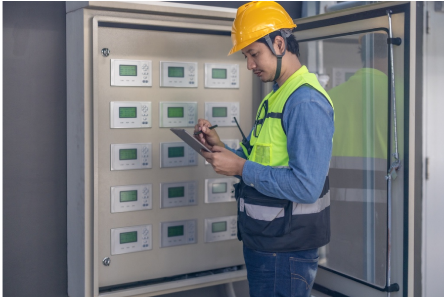
Inspection of HVAC control panel
