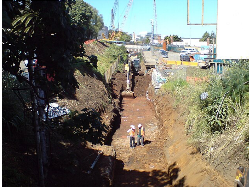
Rail corridor construction
