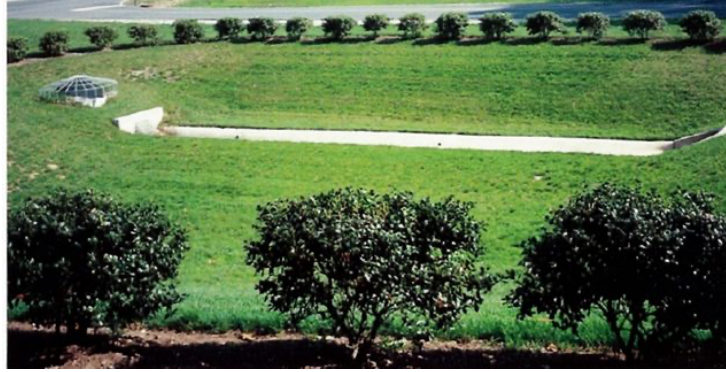
Stormwater detention basin
