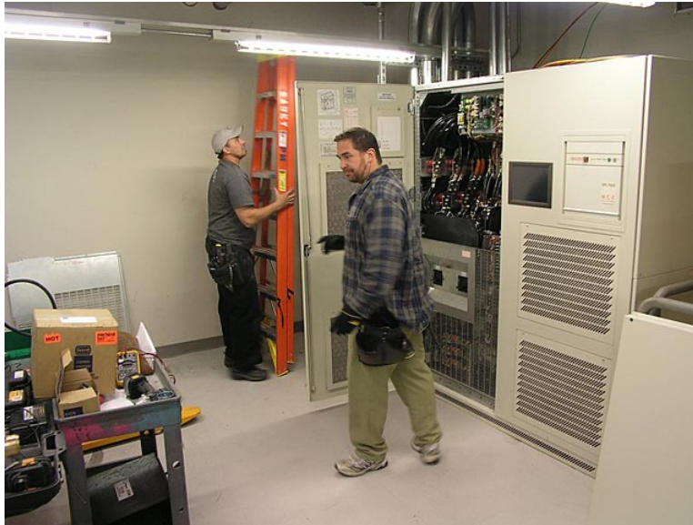
Large Uninterruptible Power Supply (UPS) being installed in a data center
