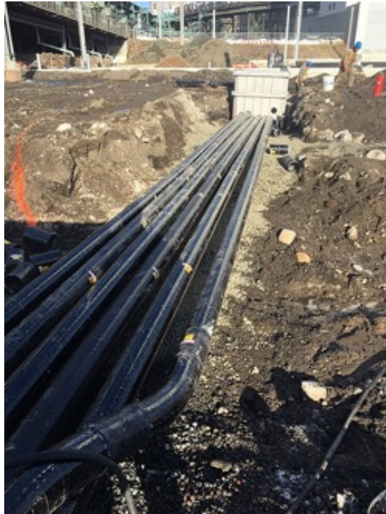
Installation of subsurface utility conduits
