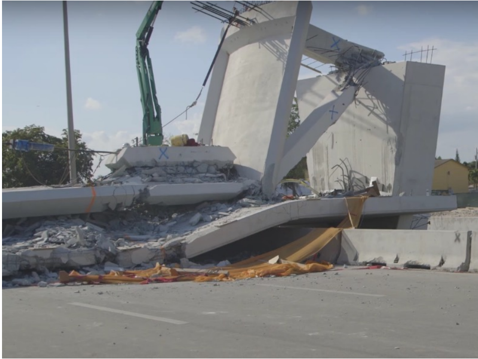
Figure 5: Florida International University bridge collapse
