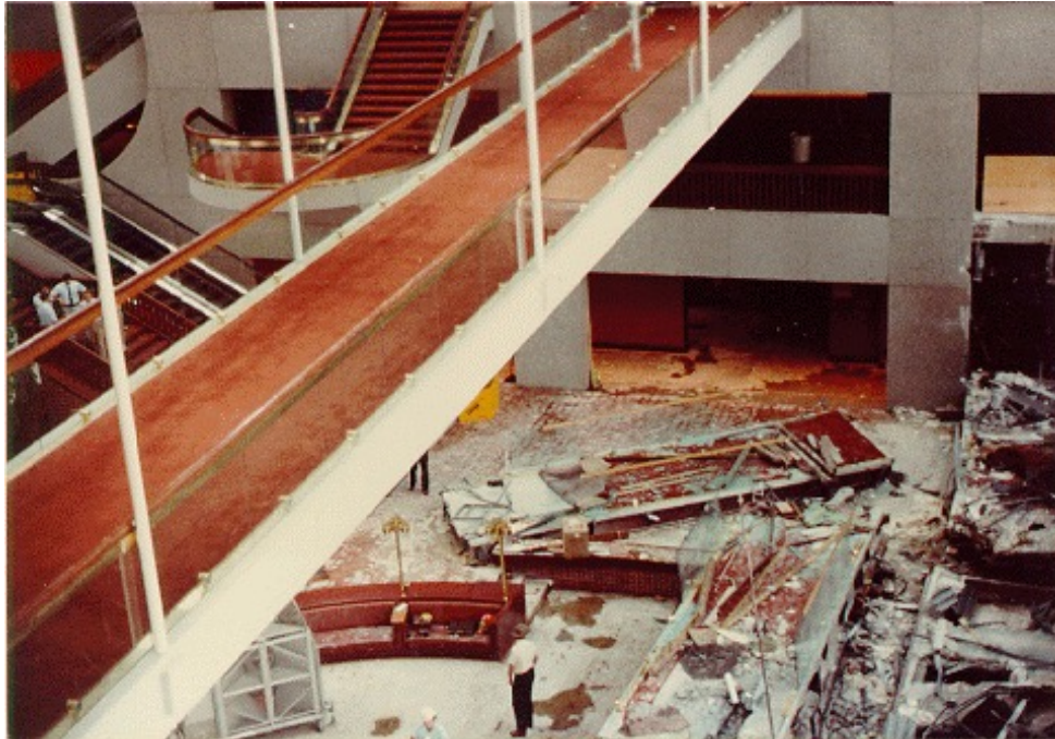
Figure 1: Hyatt Regency Hotel walkways collapse caused by the builder replacing the originally designed single-rod system with a double-rod support system without approval from engineers
