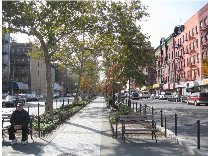
Figure 6: Wide pedestrian refuge island
