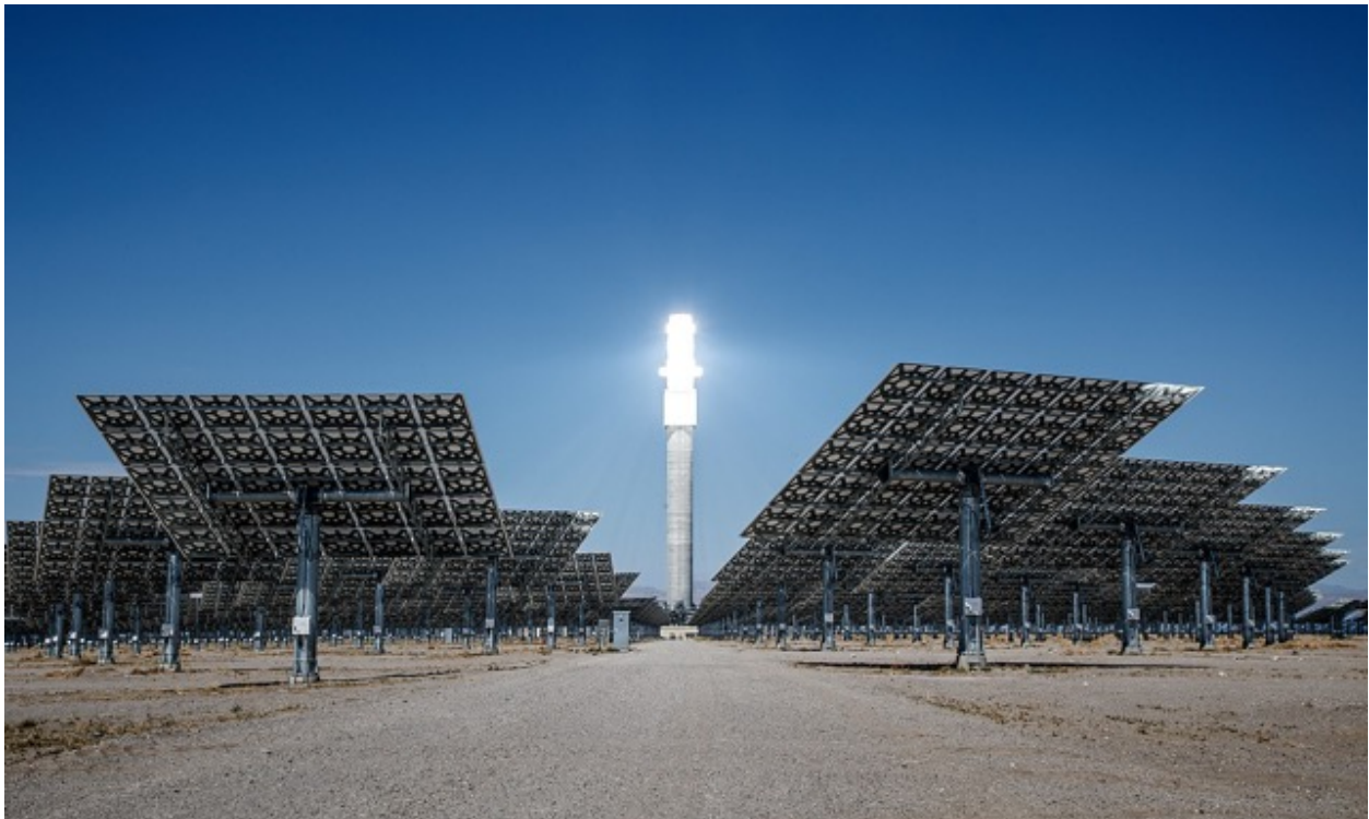
Figure 1: Solar Reserve's Crescent Dunes: Sunlight heats molten salt that flows through a 640-foot receiver tower to over 1,000 degrees, causing the top to glow white hot.
