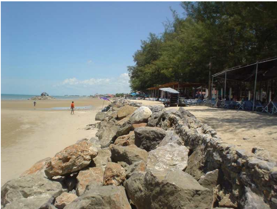
Figure 6: Seawall used to prevent can control coastal erosion
