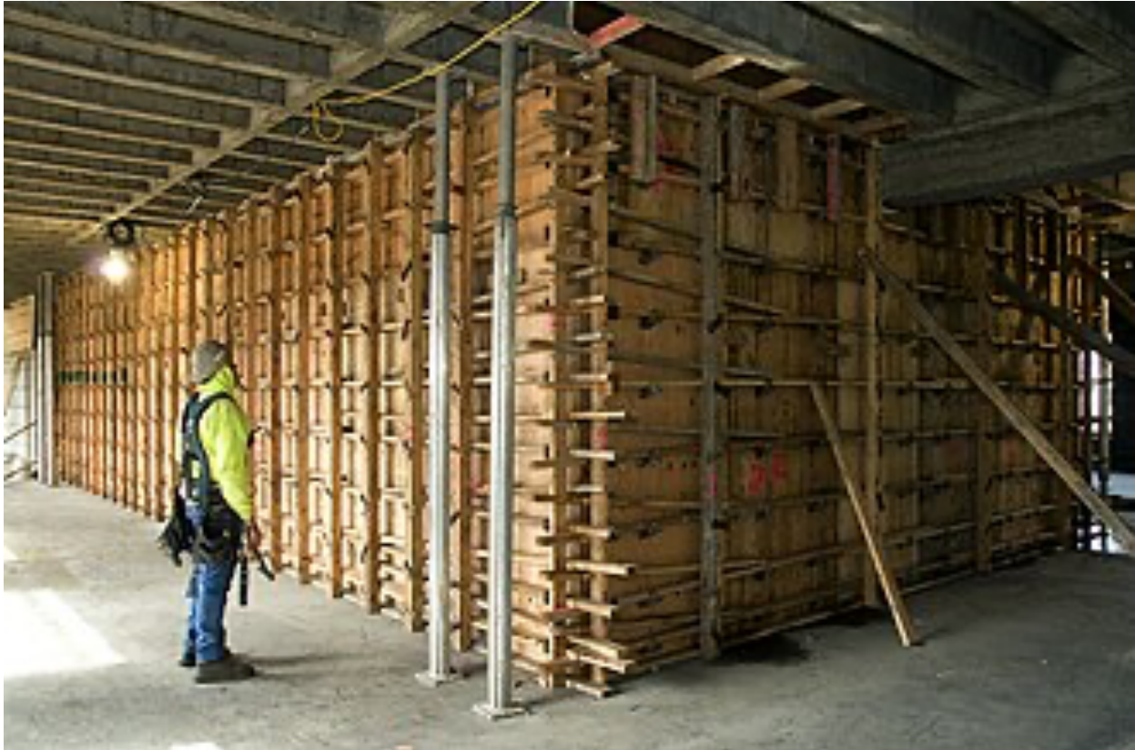
Figure 3: A construction worker inspects the frames for new shear walls that will give added structural support to the building.
