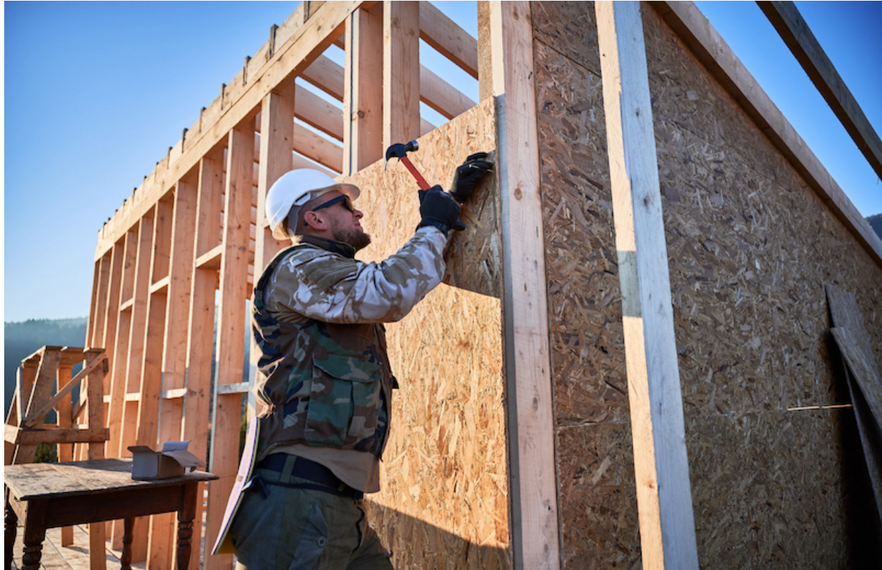
Figure 5: Oriented strand board panels nailed onto wooden frame of house.
