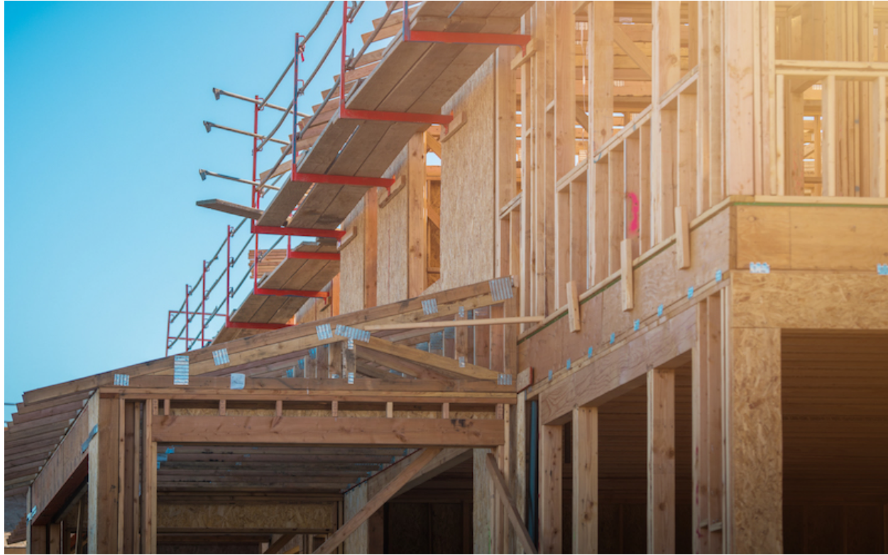
Figure 8: Shear walls in multi-story building development.
