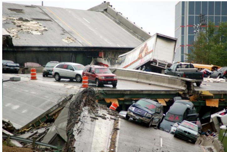
Figure 8: Collapsed portion of the I-35W Mississippi River Bridge (US Coast Guard).
