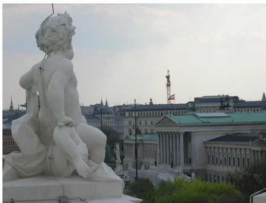
Figure 11: Lightning conductor system on Austrian Parliament building.
