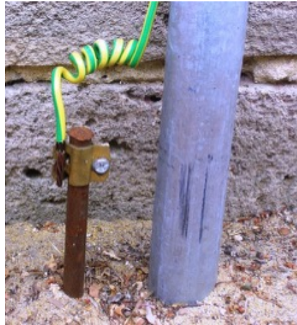
Figure 8: Typical grounding electrode.
