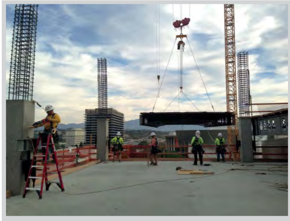
FIGURE 18 Fly table (courtesy of Charles Pankow, Ltd and Doka Forms)
