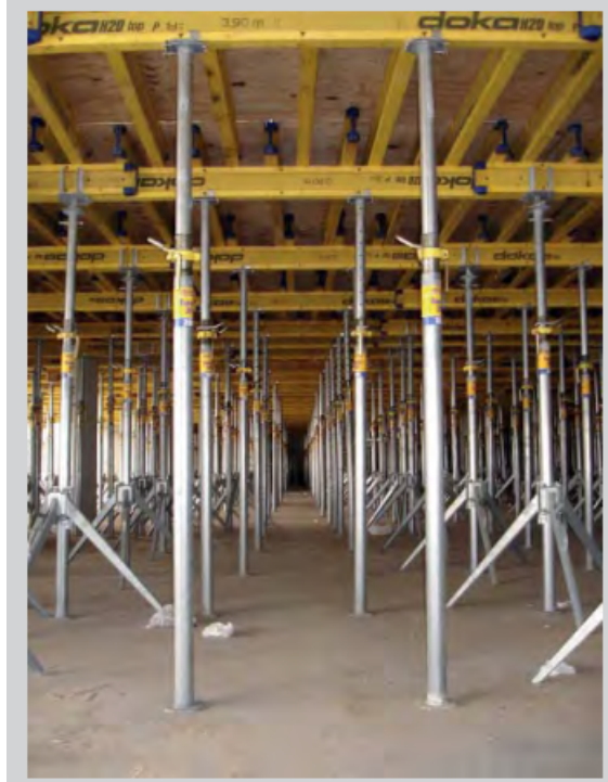
FIGURE 24- Doka form system (courtesy of Charles Pankow, Ltd and Doka Forms)
