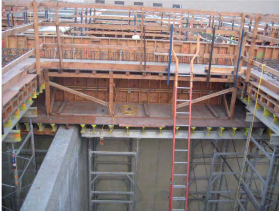
FIGURE 12 Slab and dropped beam
