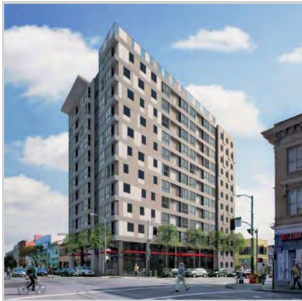
FIGURE22 - 1321 Mission Street apartment building (Courtesy of Charles Pankow, Ltd and Doka Forms).
