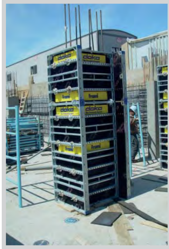
FIGURE 27- Column forms (courtesy of Charles Pankow, Ltd and Doka Forms).
