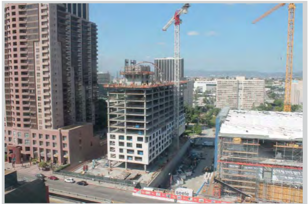
FIGURE 16 Twenty-story apartment building, Los Angeles, California (courtesy of Charles Pankow, Ltd and Doka Forms)
