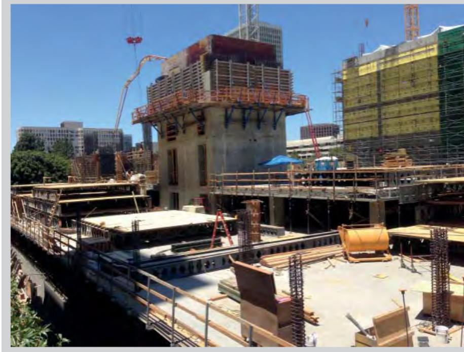
FIGURE 20 Jump form system (courtesy of Charles Pankow, Ltd and Doka Forms).
