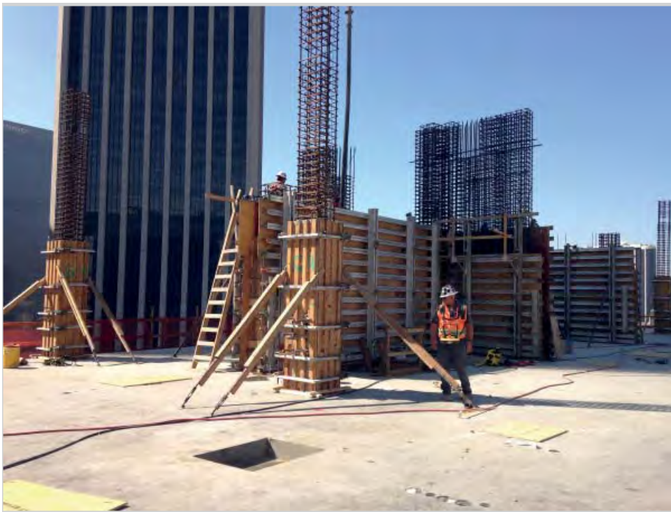
FIGURE 21 Concrete gravity columns and shear walls (courtesy of Charles Pankow, Ltd and Doka Forms).
