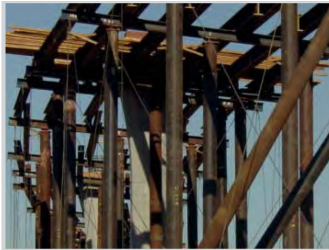
FIGURE 2- Typical falsework for this project
