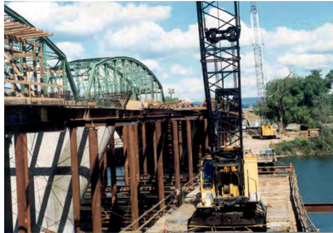
Figure 1- Pipe Post Falsework
