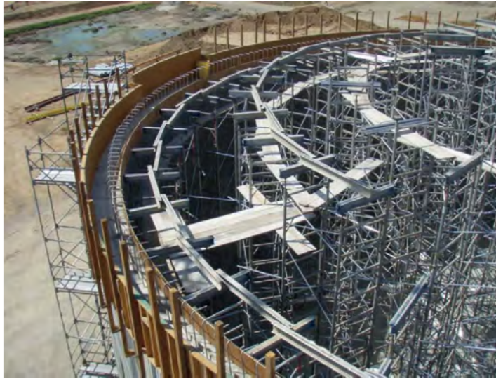
FIGURE 4 Water tank falsework using aluminum system
