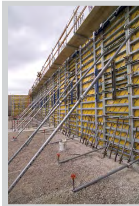
FIGURE 28- Wall forms (courtesy of Charles Pankow, Ltd and Doka Forms)
