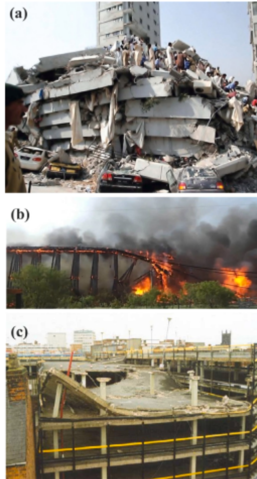
Fig. 3. (a) Pancake collapse of a reinforced concrete structure following an Earthquake in Islamabad, Pakistan , (b) Domino collapse of a wooden trestle bridge in Texas, the USA , and (c) Pipers Row Car Park partial collapse, Wolverhampton, the UK .
