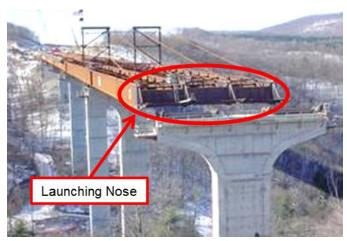
Figure 12 Photograph showing an I-girder launch with launching nose and cable tie-backs
