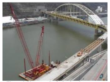
Figure 4 Photograph of a lattice ringer crane
