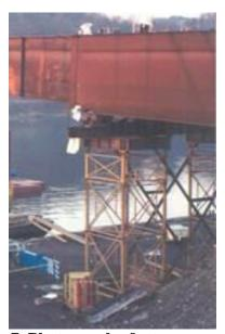
Figure 7 Photograph of a temporary bent
