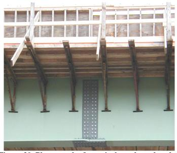
Figure 20 Photograph of a typical overhang bracket
