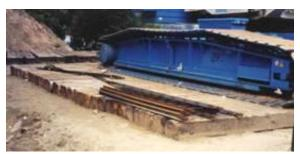
Figure 6 Photograph of a timber crane mat
