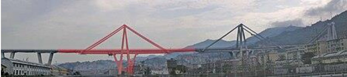
Image: (Wikipedia) collapsed segment of bridge in red
