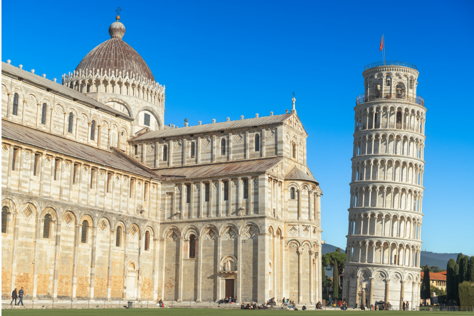
Figure 17: The Leaning Tower of Pisa
